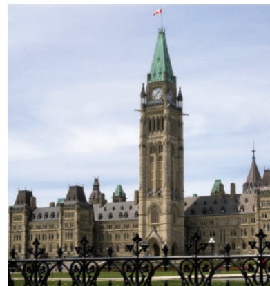
Figure 3 The green colour of copper carbonate, sometimes called verdigris, can be clearly seen on the copper rooftop of the Peace Tower at the Parliament Buildings in Ottawa.
