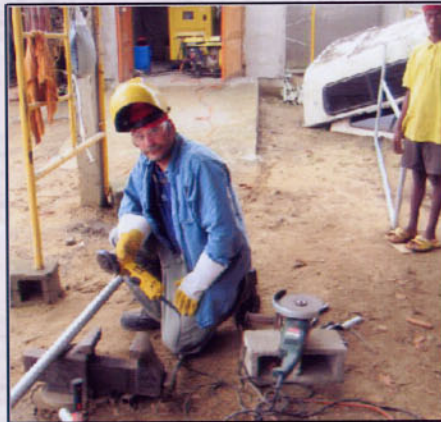
Welding the Water Tower Safety Railing
