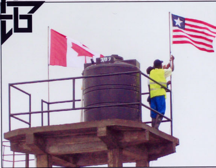
Security lightning rods as flag poles on Water Tower
